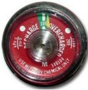
Gauge and tamper seal intact
